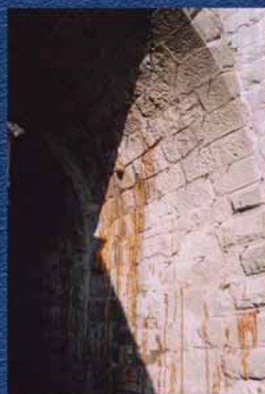
Grouting of stone bridge, reparation of bridge insulation and reinforcement
