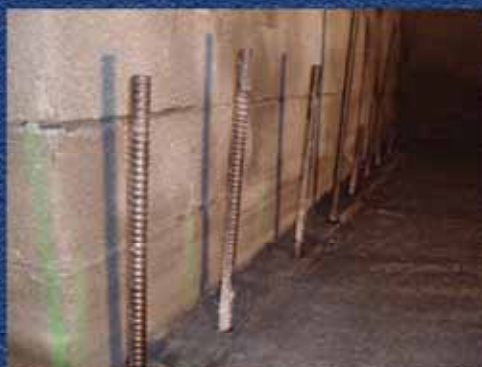
Micropiling of buildings
