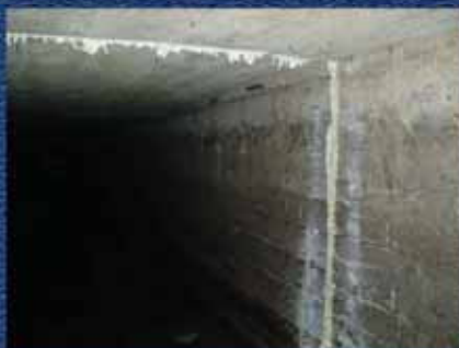
Sealing and reinforcement of the surrounding of concrete water channel under the flood dam of the Danube River near Nove Selo, Serbia, Vojvodina
