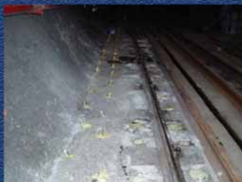
Reinforcement and sealing of concrete of subway track in Budapest
