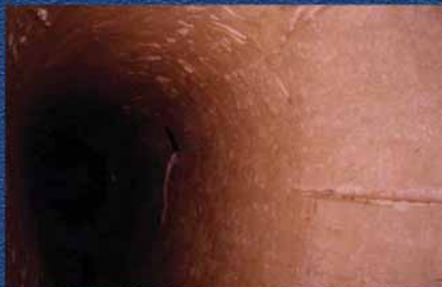
Using of polyurethane organic-mineral material for concrete sewer lining
