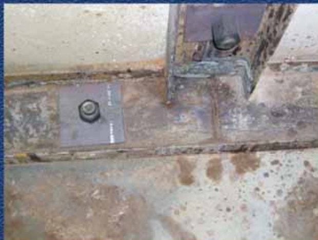
Micropiling of building foundations
