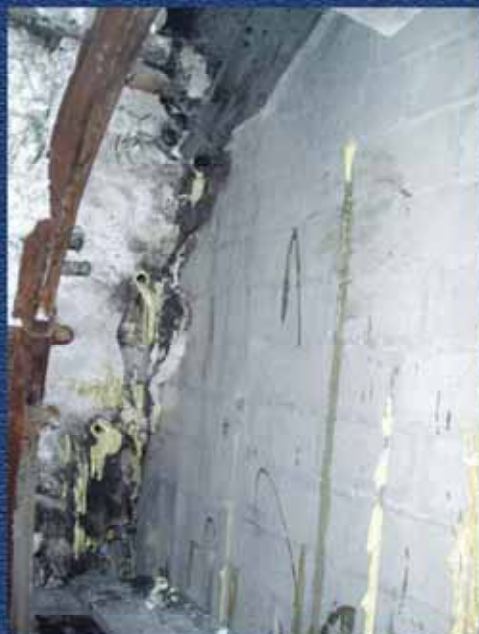
Sealing of gas emanations at the Hullera Vasco Leone mine, Spain 2006
