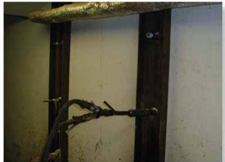
Anchoring of steel constructions and grouting of masonry
