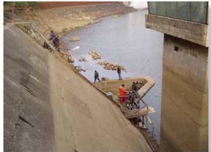
Sealing of Berdu dam in Romania
